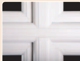
Arrissed Joints Mimicking Traditional Timber Joinery
