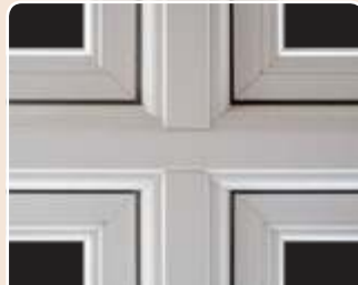
Arched Joints Mimicking Traditional Timber Joinery
