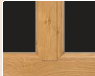
Mechanical Jointed Transoms and Mullions
