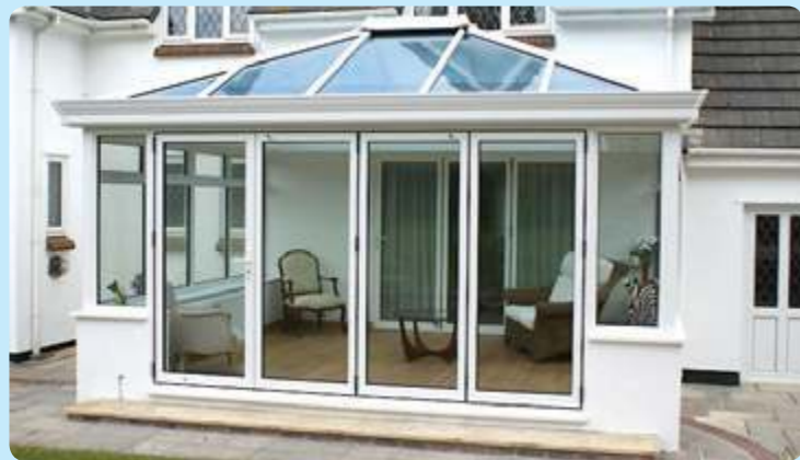
'Livin Room' orangery with aluminium frames and multifolding door
